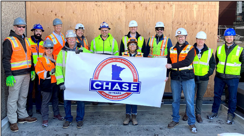
Hunt Electric Corporation and J.E. Dunn Construction • HHS Red Generator Replacement – HCMC • Minneapolis
