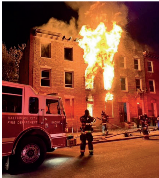
Dwelling fire in a vacant row home in southwest Baltimore City
