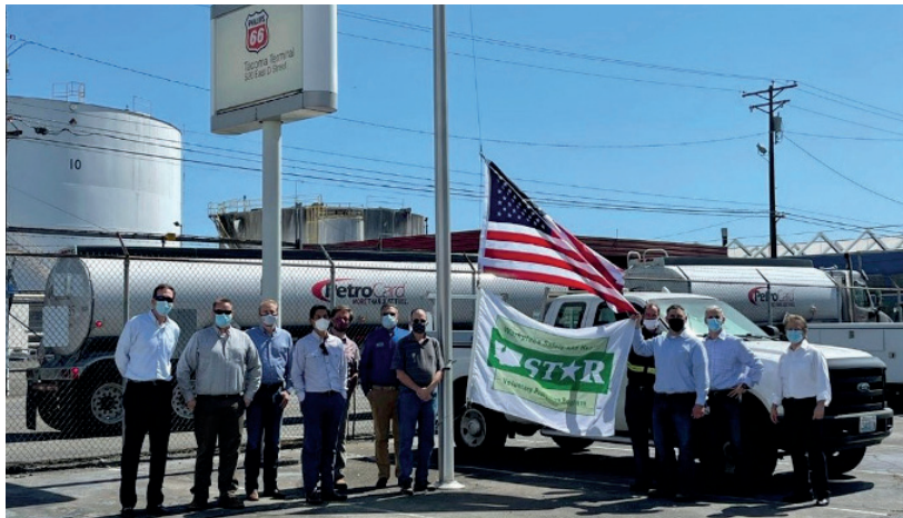
The Conoco Phillips Pipeline LLC Terminal on the Thea Foss Waterway in the Port of Tacoma, Washington
